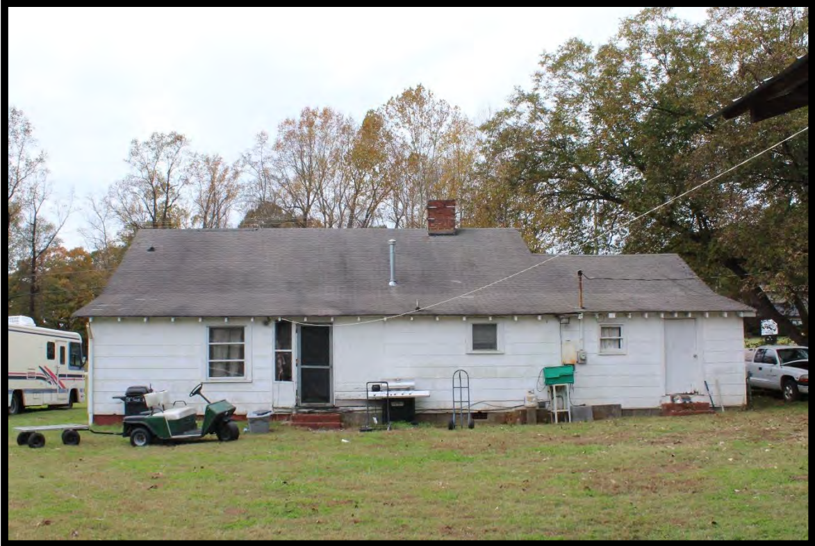
Figure 7: Chester Farmstead, Original Dwelling, Looking West.
