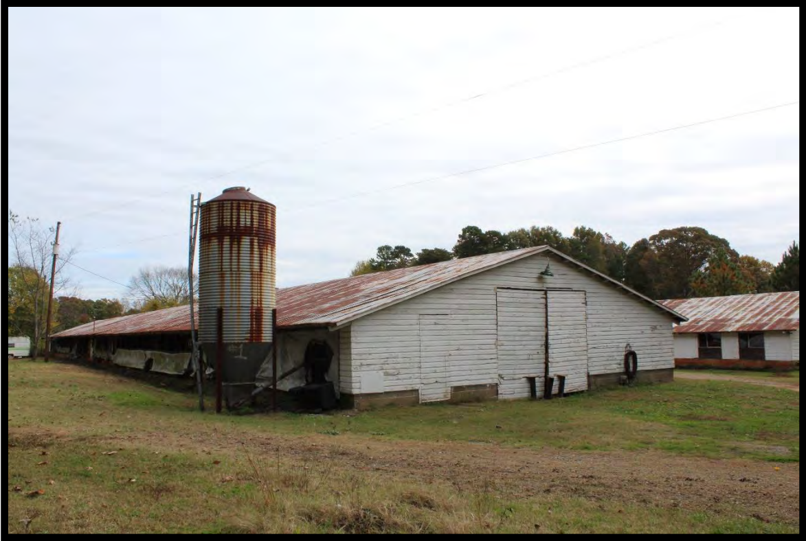
Figure 19: Chester Farmstead, Poultry Shed, Looking Southeast.
