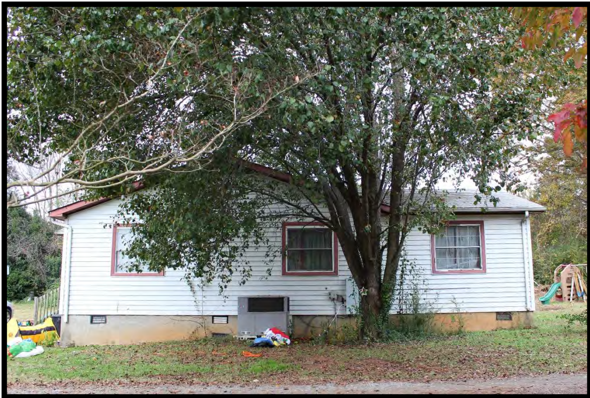
Figure 13: Chester Farmstead, Second Dwelling, Looking North.
