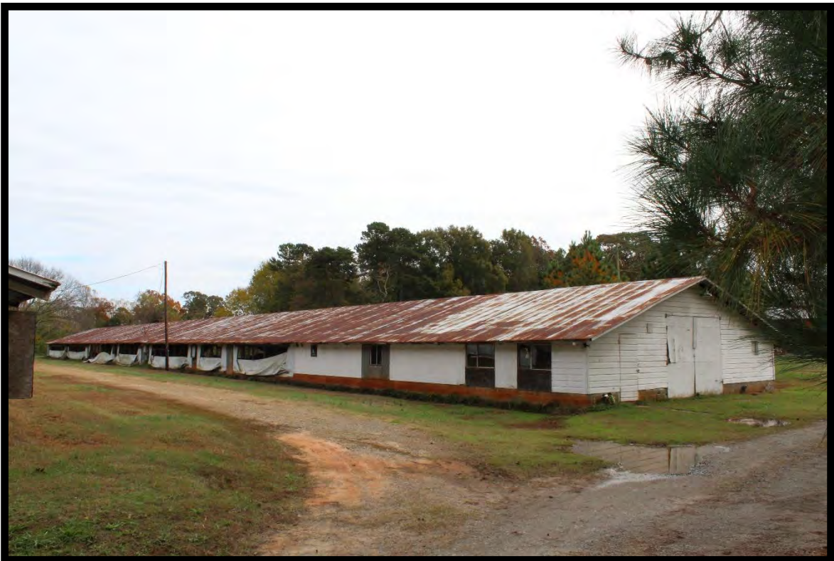
Figure 20: Chester Farmstead, Poultry Shed, Looking Southeast.
