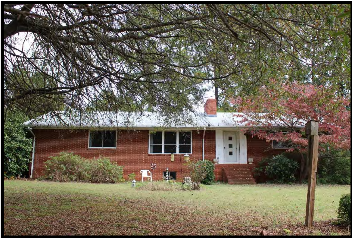
Figure 15: Chester Farmstead, Ranch Dwelling, Looking East.
