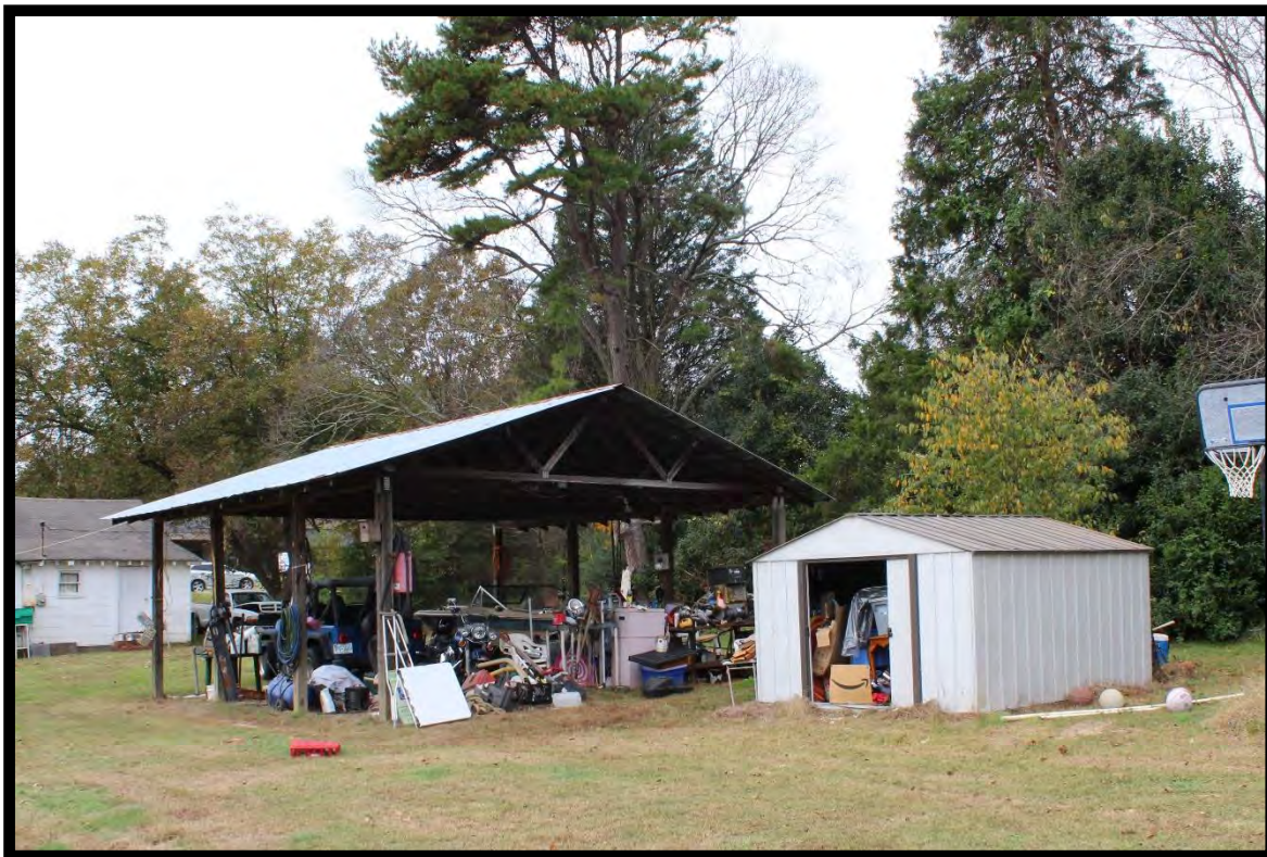
Figure 9: Chester Farmstead, Shelter and Shed, Looking Northwest.
