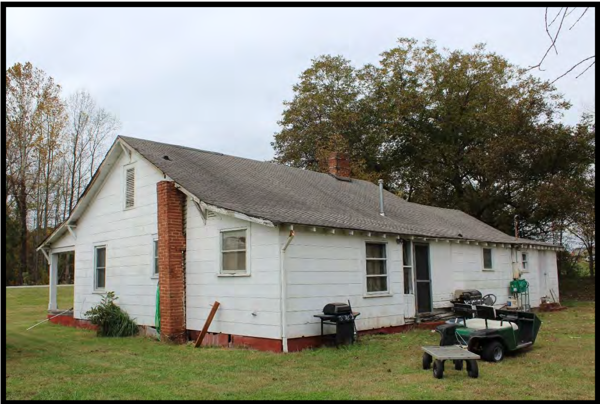
Figure 8: Chester Farmstead, Original Dwelling, Looking Northwest.
